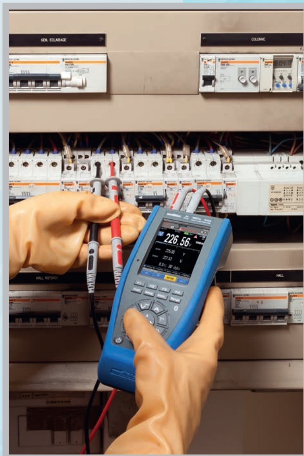
Measurements on electrical cabinets
