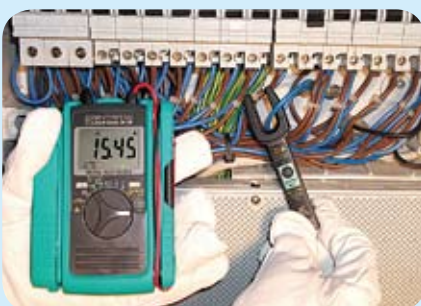
Measuring current in a Switchboard
